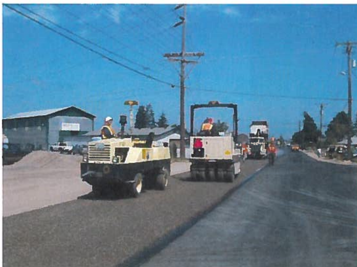
Once rock chips are applied to the liquid asphalt they are rolled in with rubber-tired rollers
